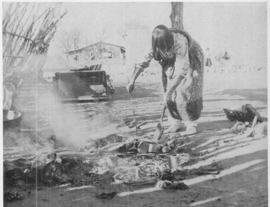
The firing finished, the improvised oven is dismantled and the pottery removed.
