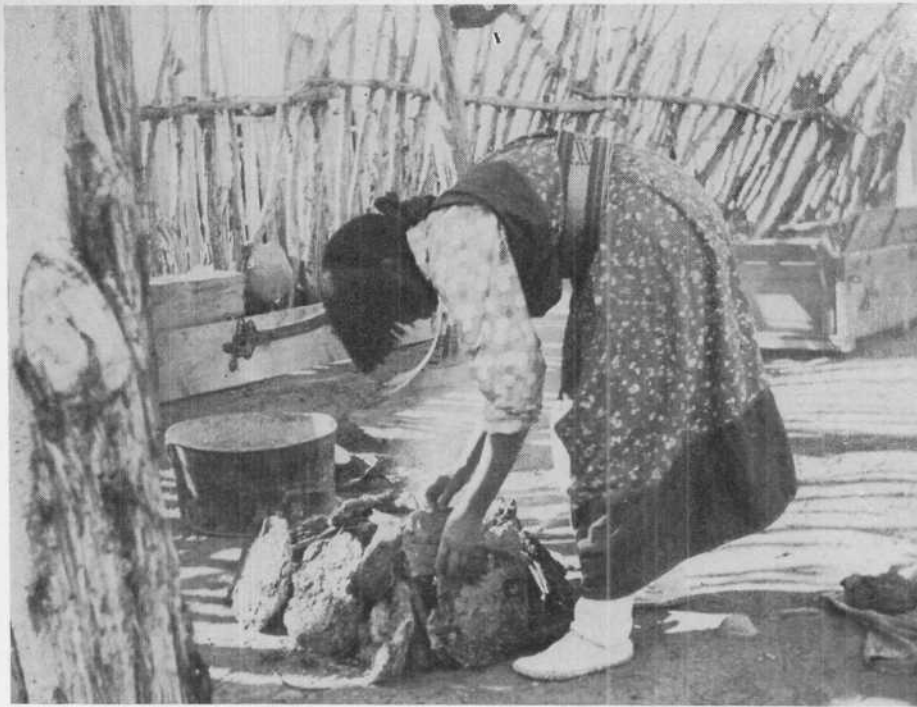
Heaping manure against the framework of the oven made of tricycle wheels and tin cans surrounding the pottery to be fired.
