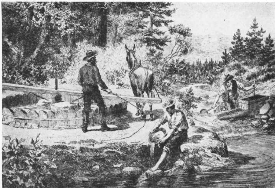
Old print showing three primitive gold recovery methods—pan, rocker and arrastre. Used by the '49ers, the gold pan and rocker are still employed today and are easily adapted by the amateur. Ruins of arrastres or drag-stone mills may be found throughout the Southwest. Photo courtesy California State Division of Mines.
