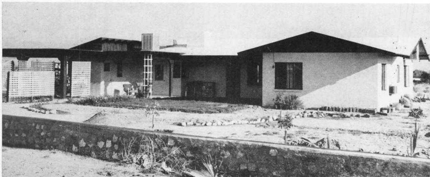
Rear view, from the southeast, with patio (in process of landscaping) and porch which will serve as an outdoor dining room. The three cooling units may be seen in this picture. On the east wall is the evaporative cooler under the cornice, and the refrigeration unit in the studio wall lower down. The second evaporative unit on the porch is not visible from the front of the house.
